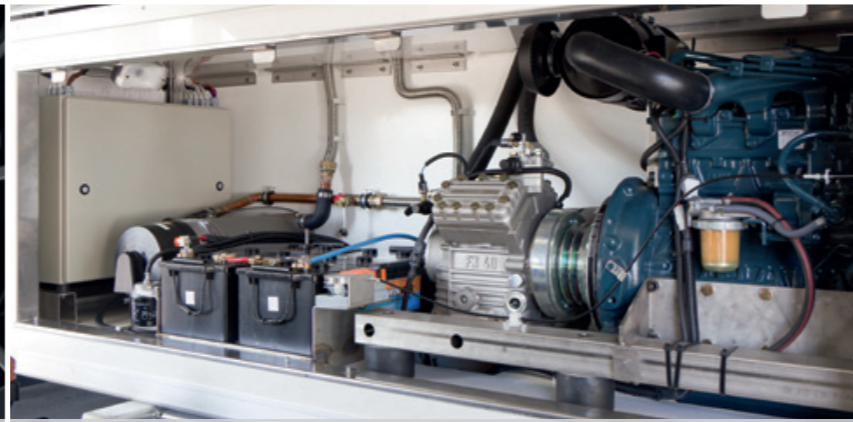
■ Three layers of protection: EcoTransport, engine and backup batteries.
